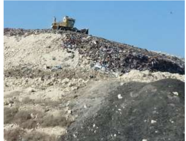
Figure 9 A photo showing the vertical expansion for the landfill
